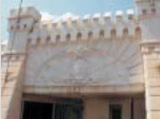
OLD FORT ENTRANCE
